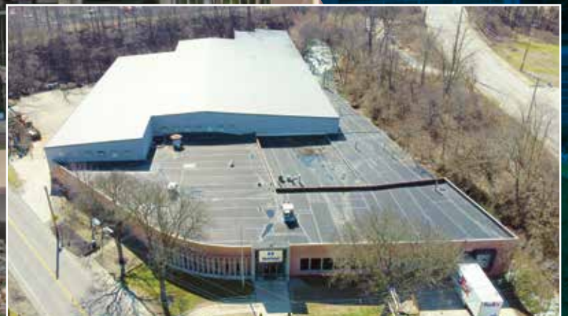
Ken-Tool's 100,000 Square Foot Akron, Ohio Facility
